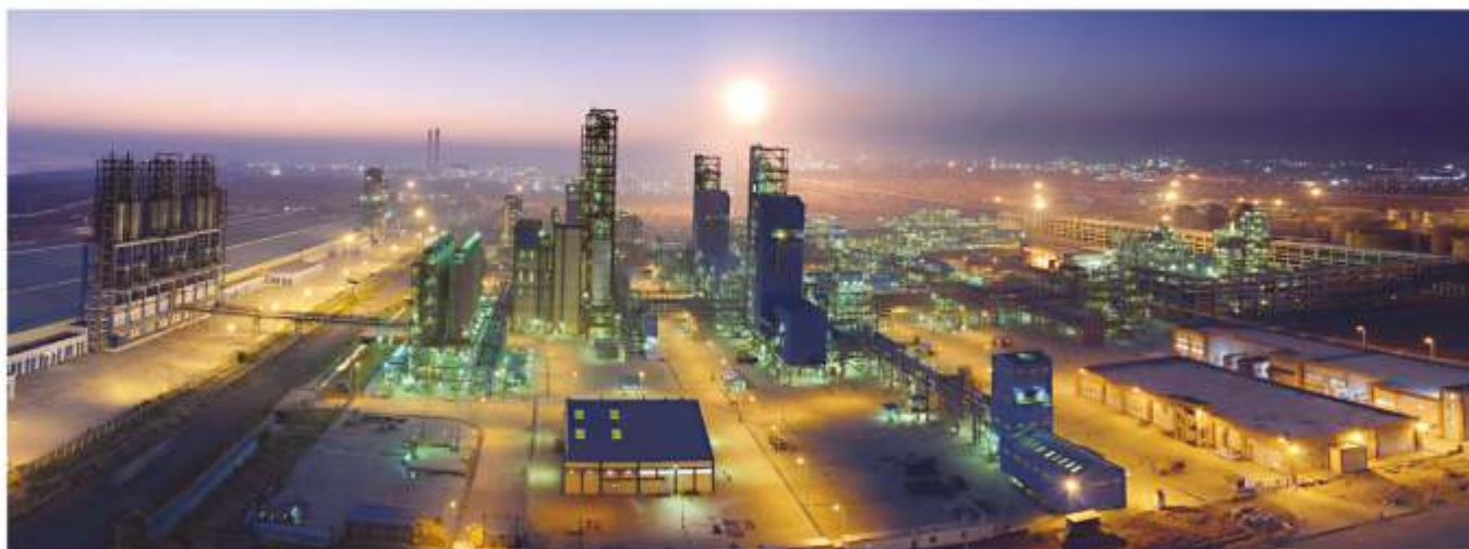
OPaL Plant's view at Dahej
